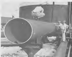
WORKERS ALONGSIDE and astride the 36-inch line indicate just how big the pipe is.
